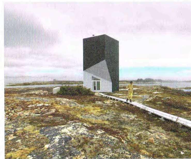
TOWER STUDIO Dramatic angles characterize this studio, perched on the rocky coastline of Shoal Bay in the island's north.
