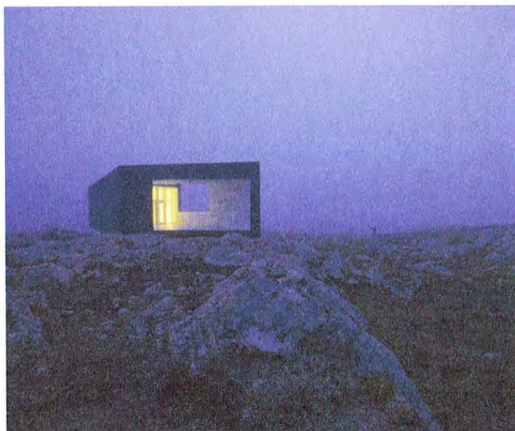
LONG STUDIO At 1,292 square feet, the studio is Fogo Island's largest, with an enclosed terrace framing the ocean view.
